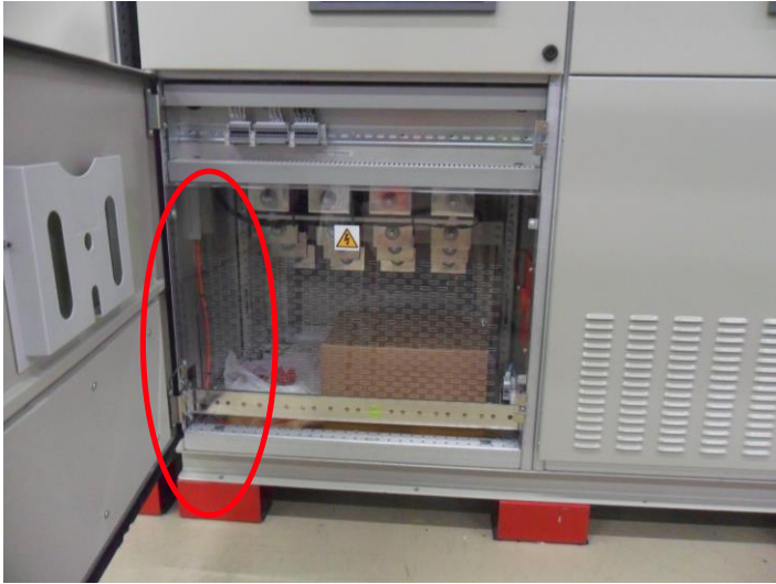
Heat Detector Cable
