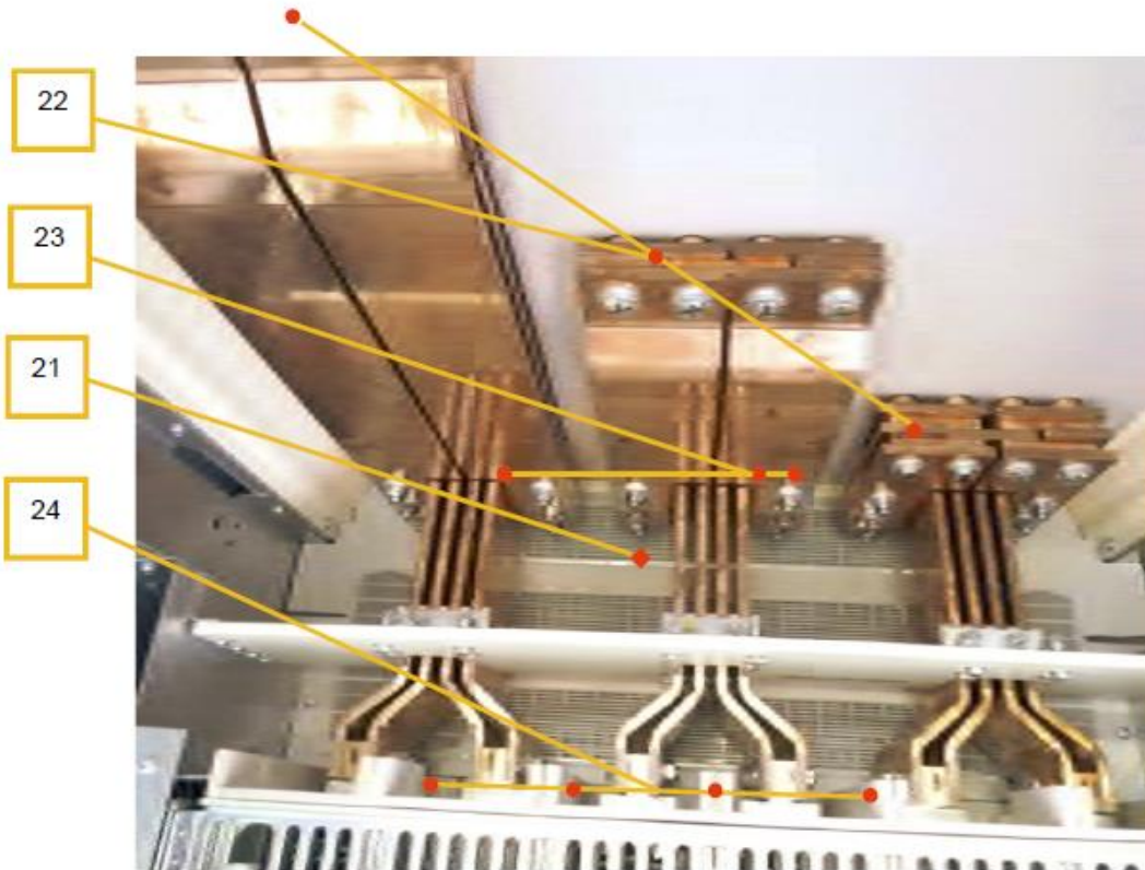
Diagram 6: Arrangement of selected temperature-measuring points in section C01
