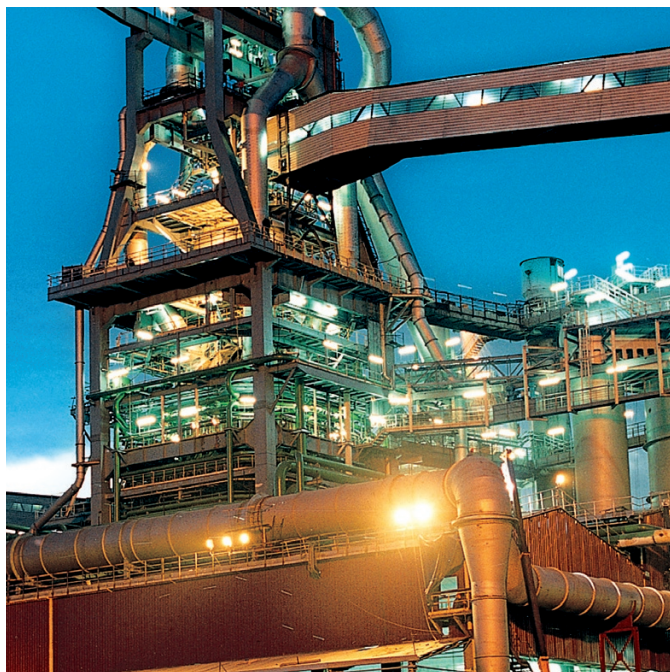
Industrial application: Refinery
