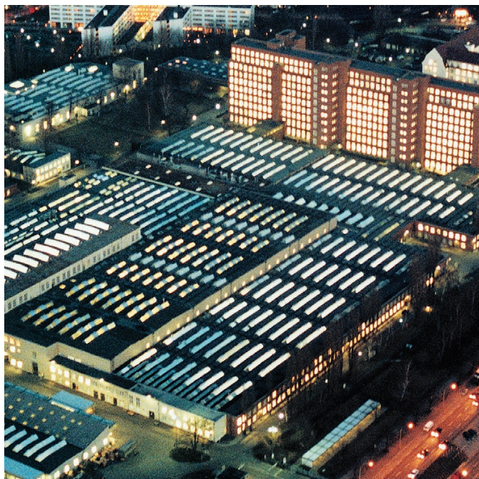
Switchgear Factory in Berlin, Germany
